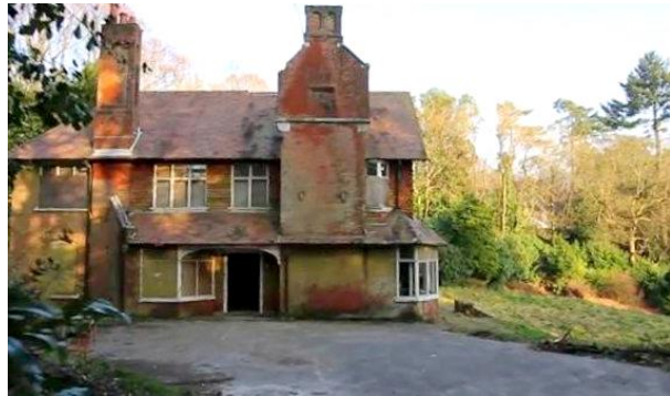
West elevation showing existing front door
